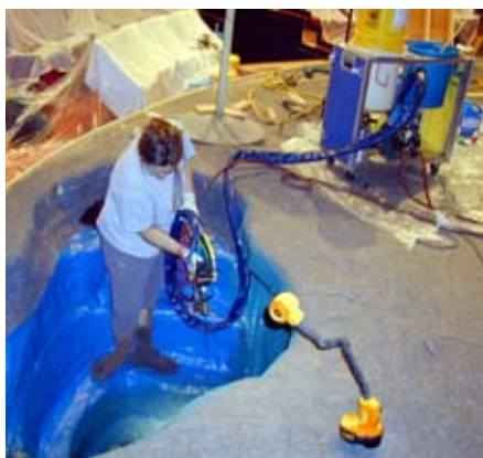
Spray Styrocoat® plastic to coat foam for theming & special effects.
