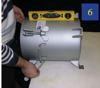
6 Make sure the chamber is level from front to back.
