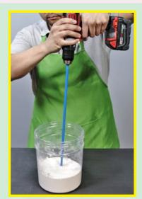
Alternatively, you can mix the material using a turbine mixer and drill. Dispense the LiquiStone™ from the bag into a seperate mixing bucket and add water.
