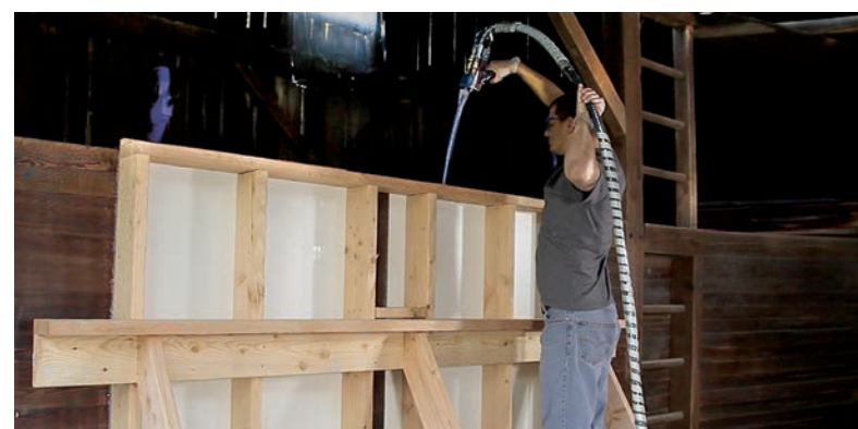
2 Mold Star® 30 is dispensed, quickly filling the gap.
