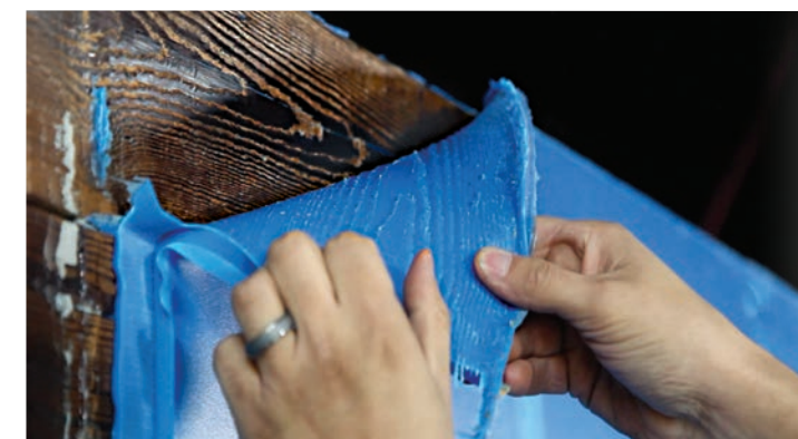
3 Cured Mold Star® 30 silicone is demolded easily from the granary wall.
