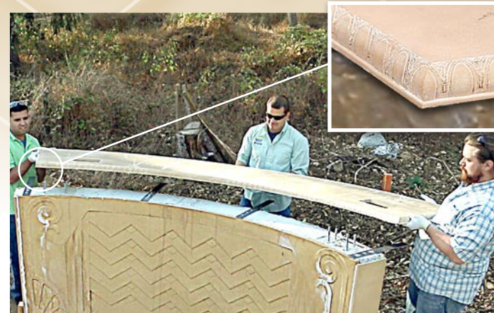
9 Custom countertops are fabricated and secured to the permanent base.
