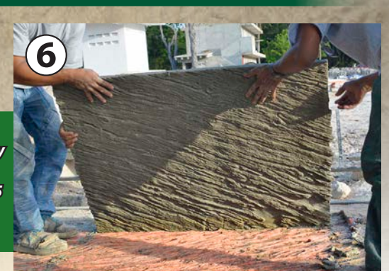
Once cured, the panels are easily removed from the Rebound® 25 mold, reflecting perfect detail.
