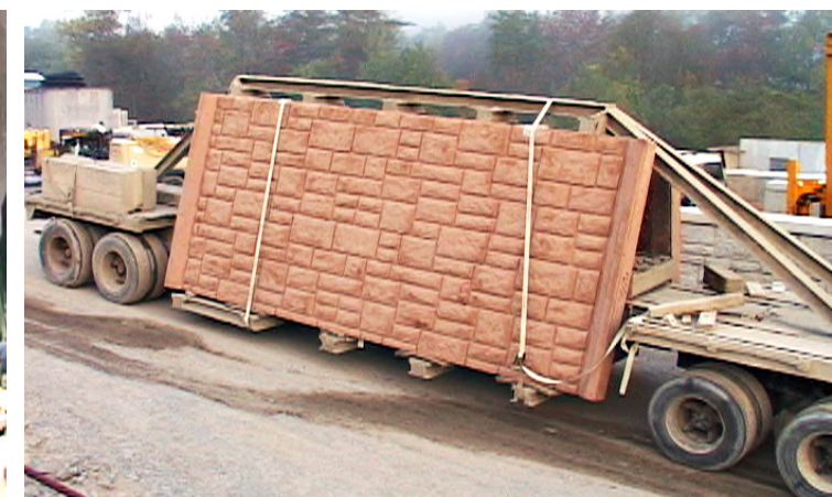
8 Completed panels are shipped to the job site.
