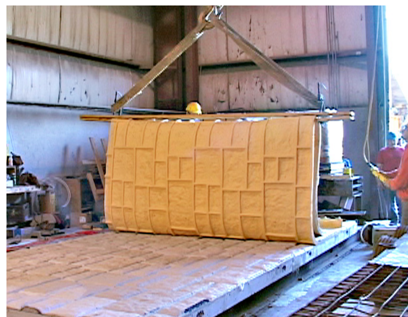
3 A power hoist is necessary to handle the 1,000 lb. (454 kg) liner.
