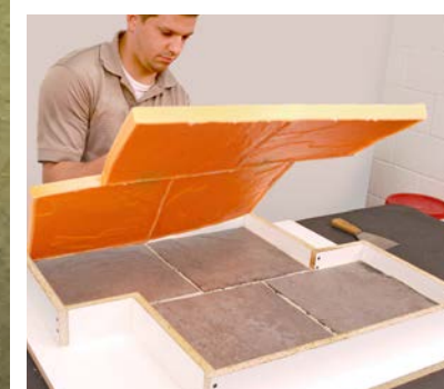
5 Once cured, stamp is demolded. Multiple stamps are made for a single job.
