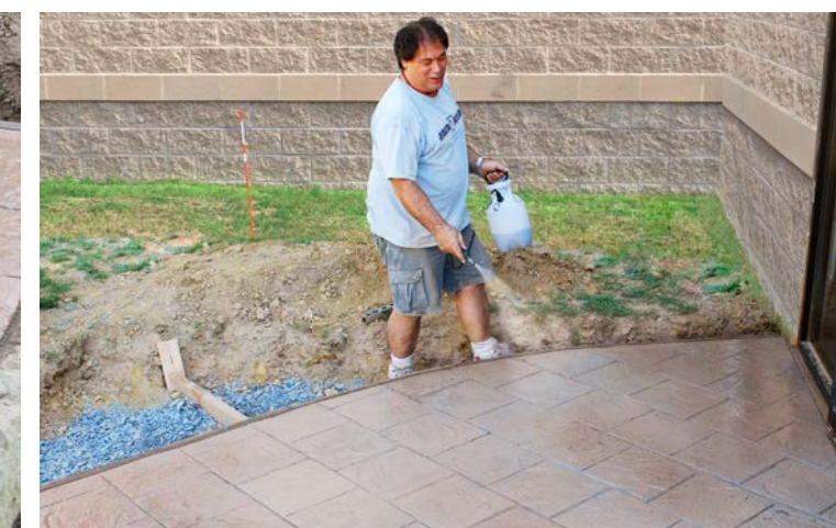
10 The concrete slab is stained and sealed.
