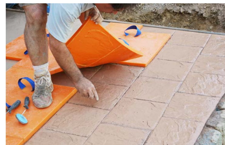
9 Stamps are then removed revealing the imprinted tile texture.
