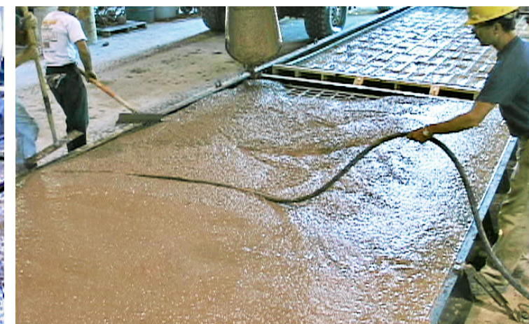
6 A drop-in vibrator helps to eliminate surface voids.
