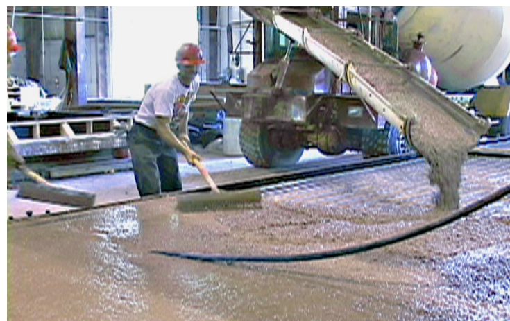
5 Concrete is poured into the mold. VytaFlex® offers excellent resistance to compressive loads without distorting.
