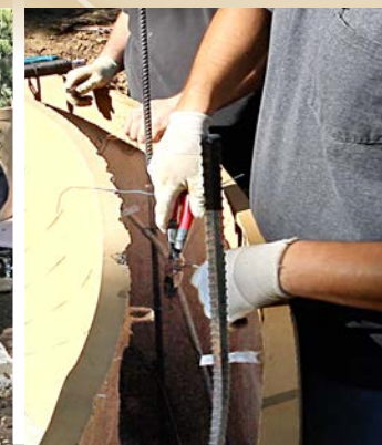
7 Precast panels are placed onto footers and fastened using anchors and rebar.
