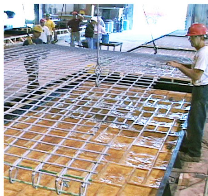
4 Rebar is positioned.
