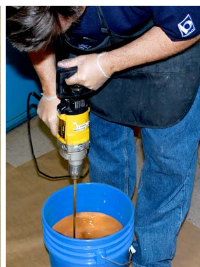
3 PMC®-780 is pigmented and drill mixed.
