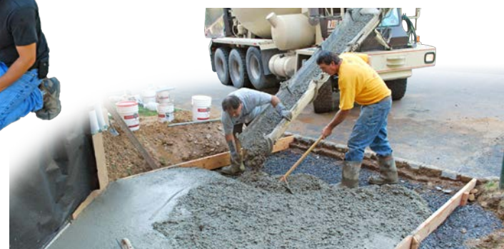
6 Ready Mixed concrete is poured at the job site.
