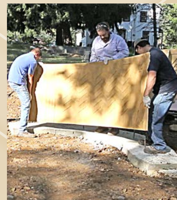
7 Precast panels are placed onto footers and fastened using anchors and rebar.
