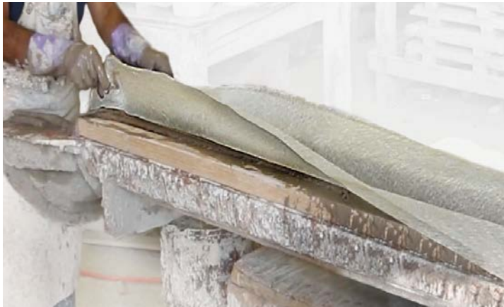
2 Once the facecoat has partially set, E-glass veil is applied.
