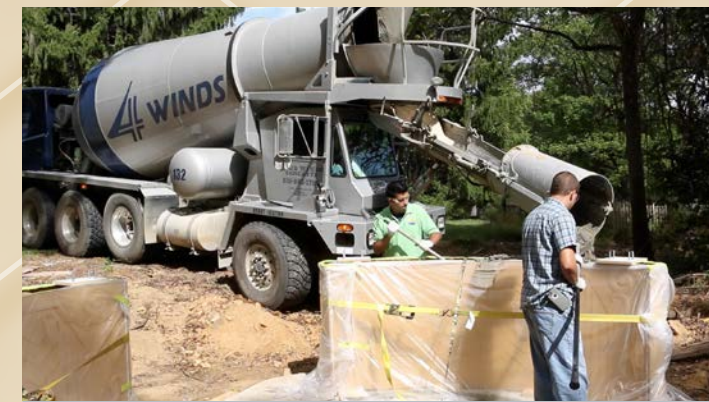
8 Ready Mixed concrete is then poured into the formwork.
