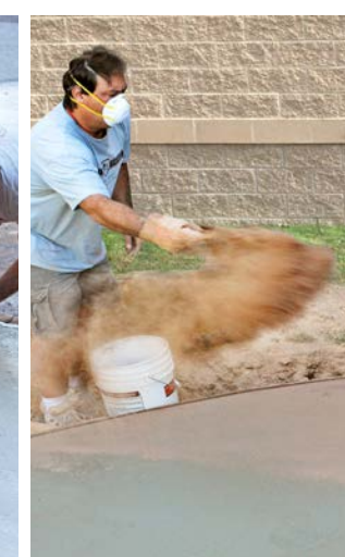
7 Concrete is screeded and color hardener is applied prior to stamping.
