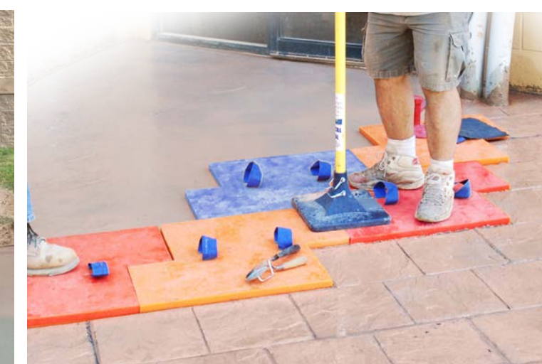
8 Stamps are positioned and hand-tamped to imprint the pattern on the concrete slab.
