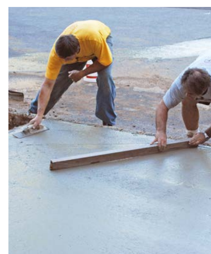
7 Concrete is screeded and color hardener is applied prior to stamping.
