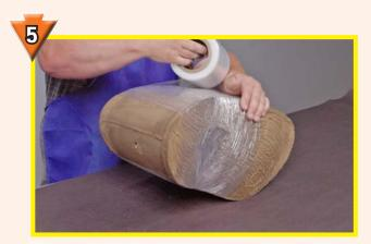
Wrap plastic film tightly around the entire area to be repaired.
