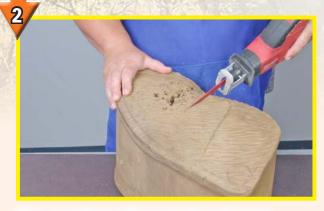
Use a reciprocating saw to cut away damaged and loose foam from the core.
