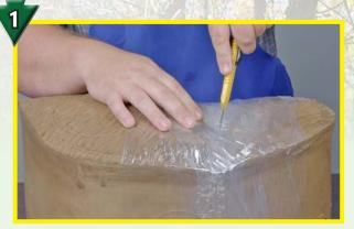
Cut a pour hole over the area to be repaired with a breakaway razor utility knife.
